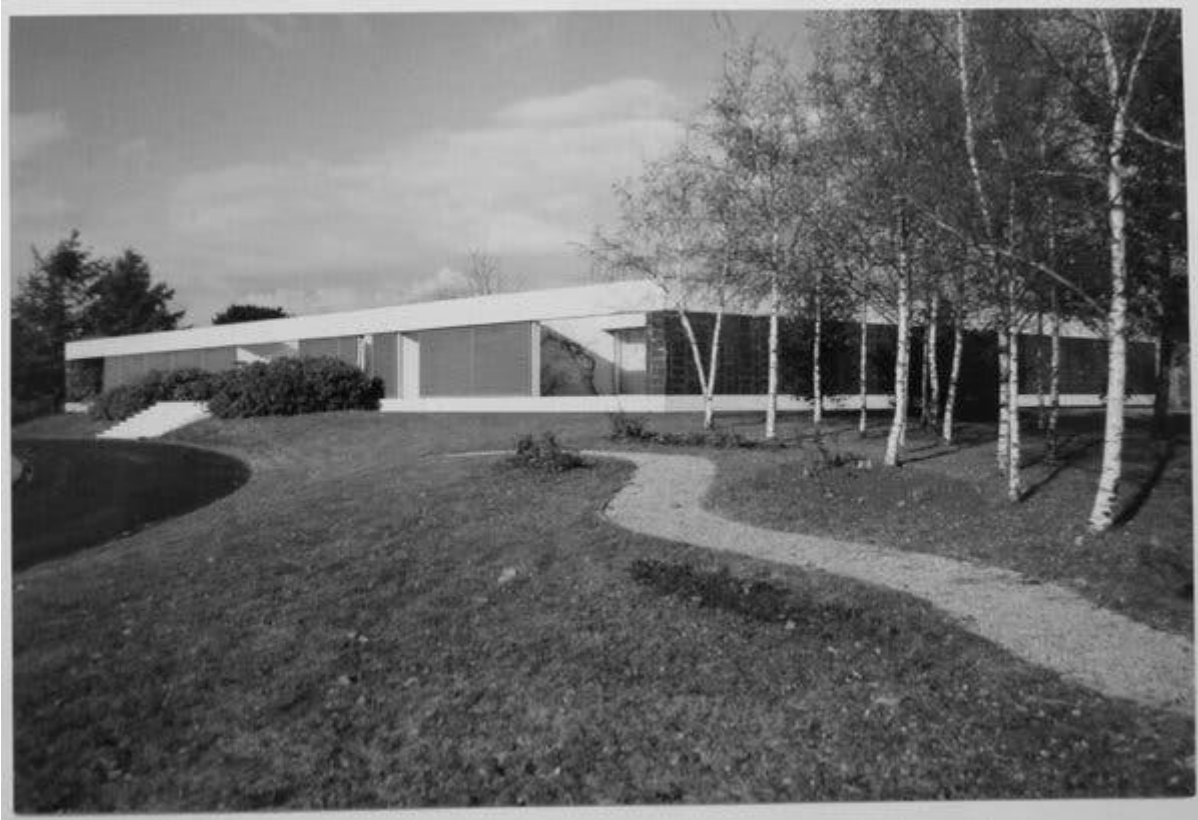
The back of Villa Weil at Domaine de Frapotel, 1980s. Terraces built within the frame of the house double as sun breaks partially protecting the glass walls of the main living spaces. Fonds Dubuisson, via SIAF/CAPA/Archives d'architecture contemporaine
